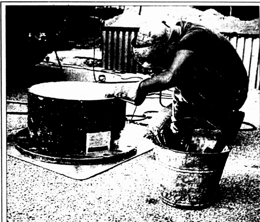
HERALD photo: Roger Cline Ray Kemper of Phillips Fabrication Inc. in Big Spring welds a flange onto a 20-inch connector pipe. Work crews were replacing a valve in a water main at the intersection of Baylor and Kentucky Way earlier this week.
