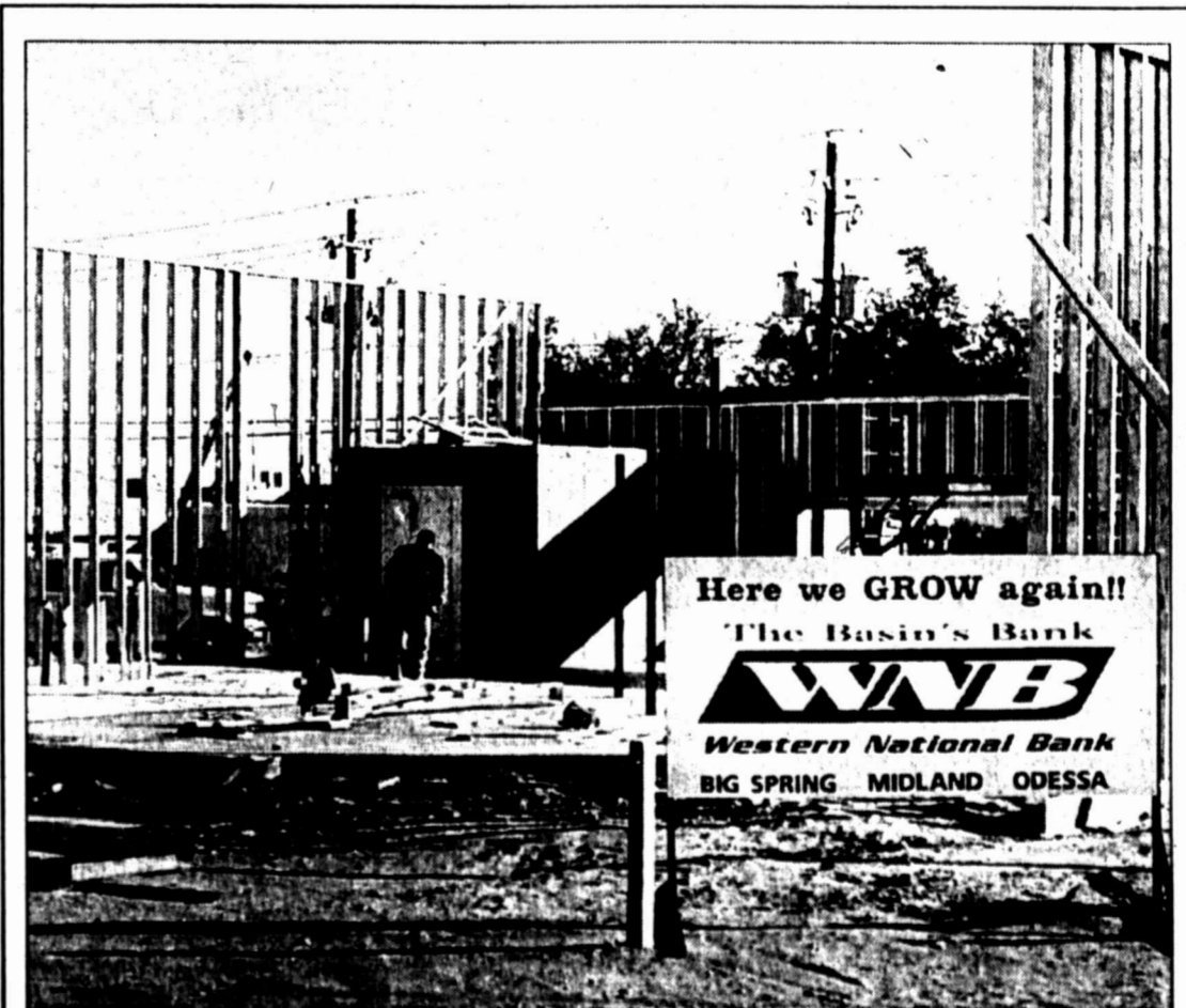
HERALD photo/Roger Cline Building a bank — Construction workers have the slab and the vault in place and are working on the walls of the new Western National Bank Branch in Big Spring. N.C. Sturgeon Construction is the general contractor on the branch, located on the corner of Scurry and Seventh streets. The branch is scheduled to open July 1.
