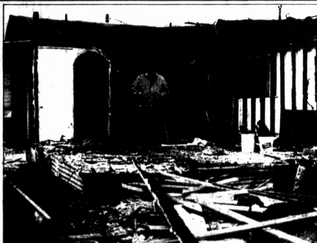
HERALD photo/Roger Cline Retired carpenter Hank Williamson stands in what used to be the living room of his home. The converted trailer home was gutted by a fire Tuesday morning. Williamson said he's grateful no one was injured in the blaze — Williamson, his wife Sandy and their two grandsons were sleeping when the fire broke out — and said the family plans to live next door with his mother.
