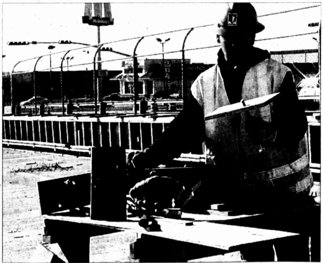
HERALD photo/Lyndel Moody Oscar Vega of Reese Construction works on erecting the new turnaround on the Gregg Street overpass. The $1.66 million project is expected to be completed by the end of this month. The project includes creating a new exit ramp on FM 700 and the turnaround.
