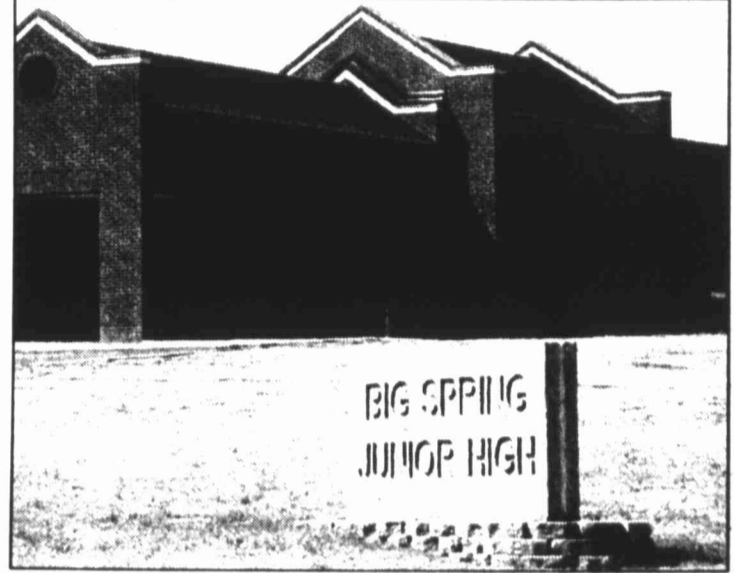
Big Spring Junior High School began developing cracks in the walls and floors soon after the facility opened in 1999.
