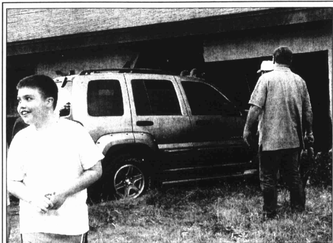
A driver reverses this Jeep Liberty from the wreckage of a house in the area of 15th and Mesa Wednesday evening after a woman accidentally drove the vehicle into the side of a relative's home. No one was injured in the accident.
