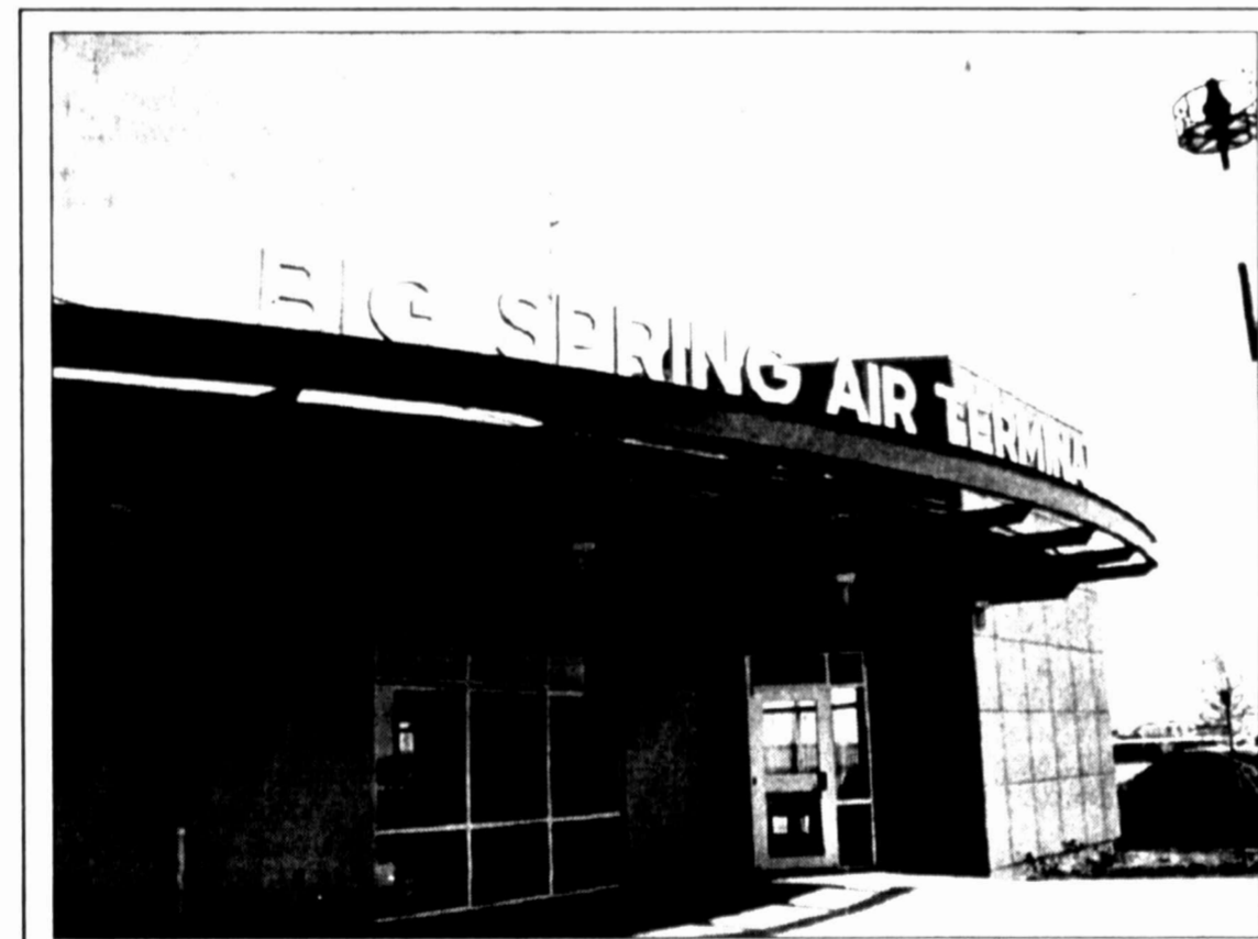
McMahon-Wrinkle Airpark Operator Nelda Reagan oversaw the building of this new airport terminal during her nine and a half years of service. Reagan resigned her position Monday, citing a desire to relax and focus her attention on her son, an Army sergeant serving in Afghanistan.
