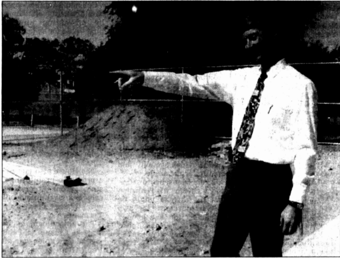
Pete Thiry, executive director of the YMCA, points out the bike hills currently under construction at the skate park. The park is expected to be completed by June 15 and will include obstacles for rollerblades, skateboards and bicycles.
