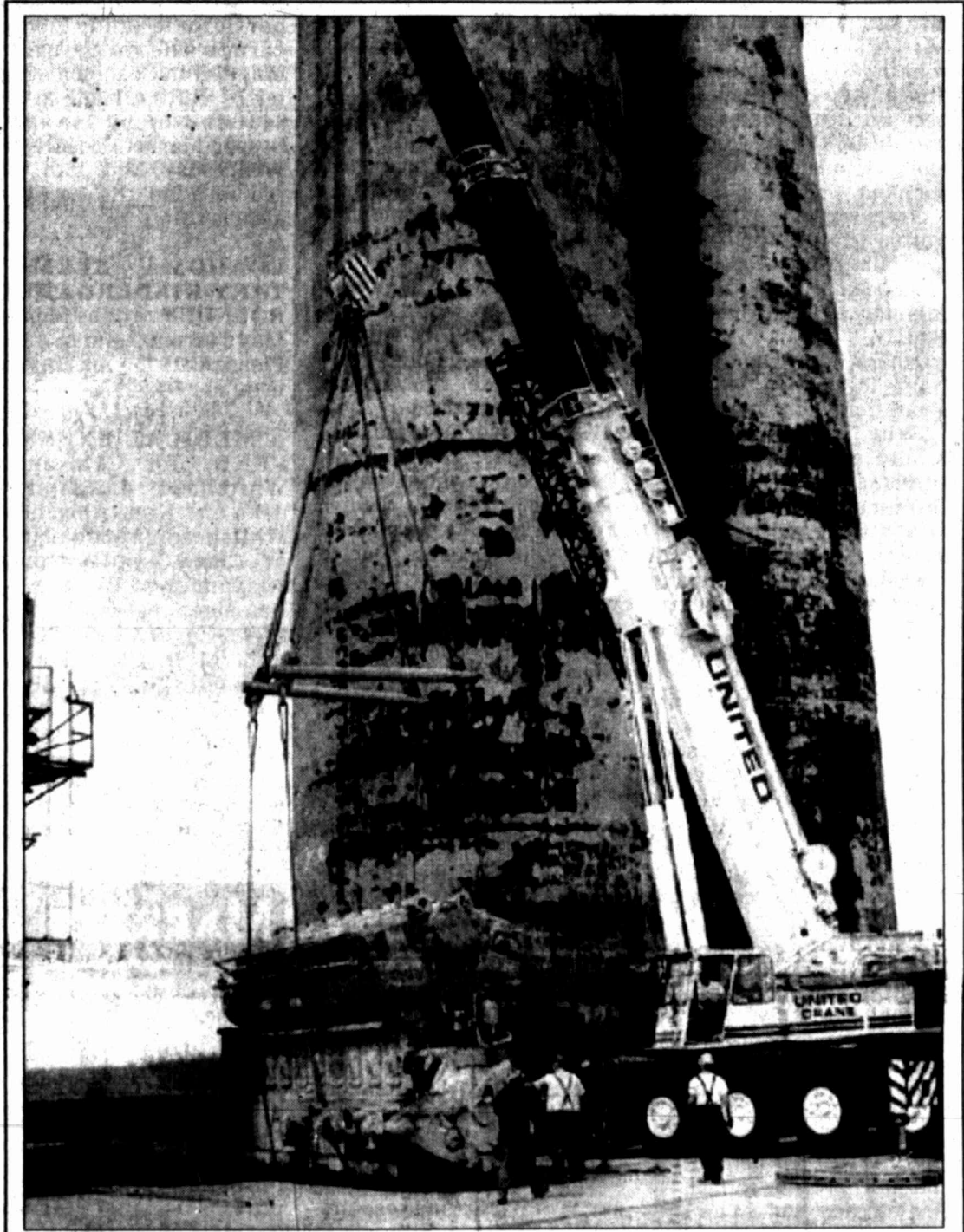
Crew members of United Crane of Houston guide this 227,000-pound electric generator onto a railroad car. TXU Electric is sending two generators to Alberta, Canada. Each generator has 4,450 horse power.
