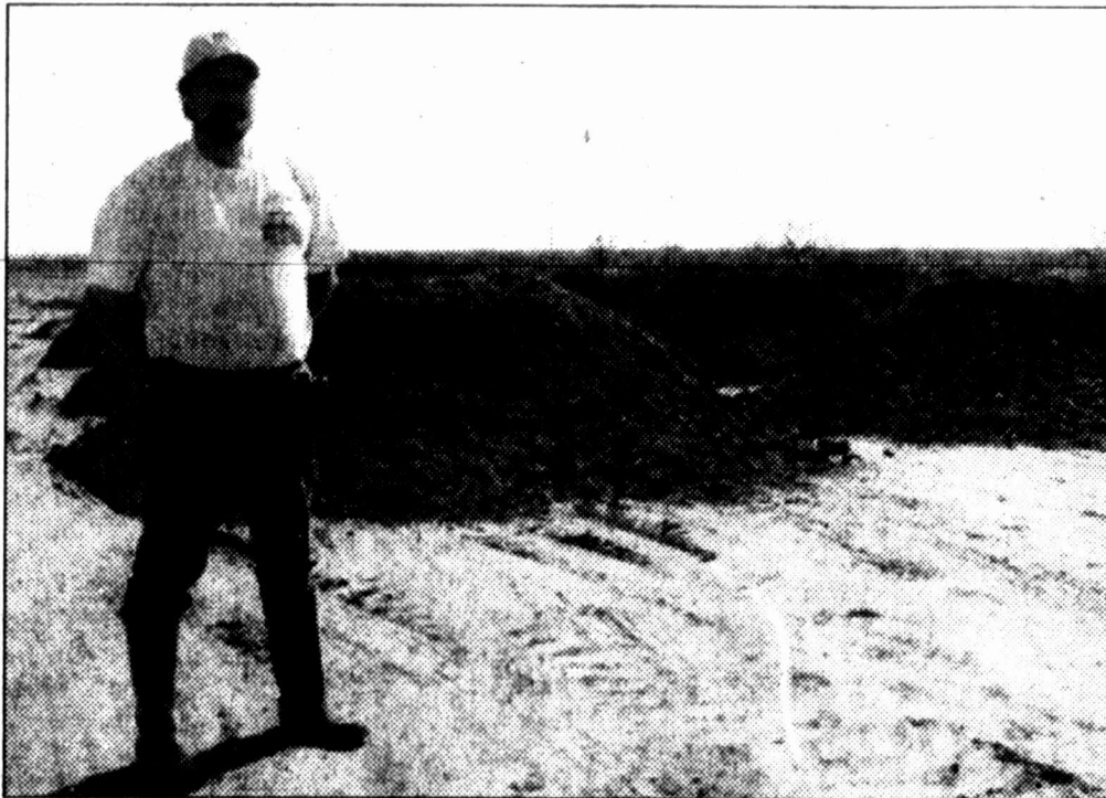
At left, James Levings, assistant manager of the Circle Six Ranch Baptist Camp, stands near piles of dirt that have been moved in preparation for construction of a new gymnasium. The project is one of several planned in coming months, thanks to growing use of the camp by church organizations throughout the area. Below, left, dirt work has also begun on a set of 16 motel-type rooms. Below, a box in the front office collects donations for the renovation project. At bottom, an artist's drawing of the planned conference center.
