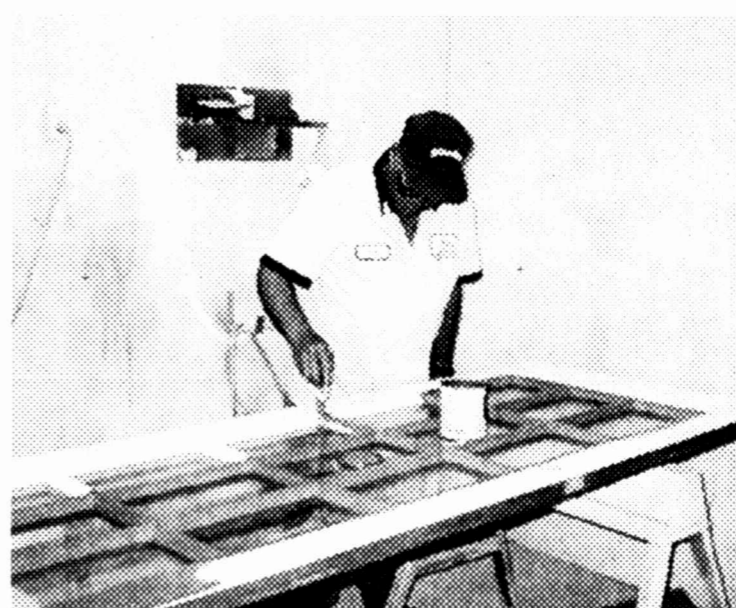
Door being painted
