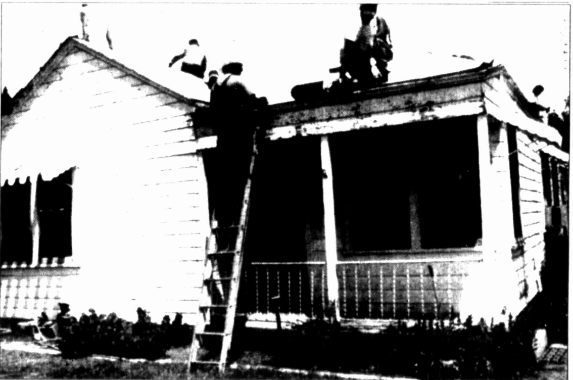
Courtesy photo A crew from First United Methodist Church installs a new roof on a home during the 2000 Christmas in April workday. This year's workday is April 28, when hundreds of volunteers are expected to join the effort to repair homes for the elderly, low-income and handicapped.
