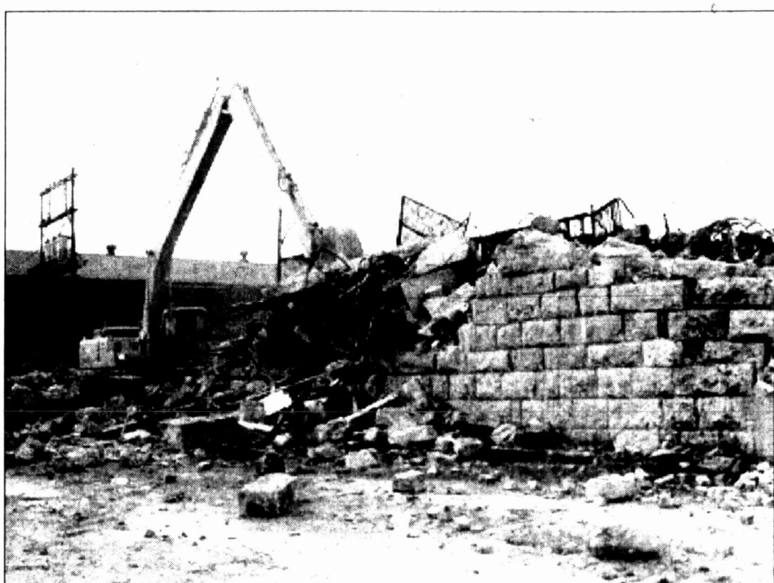
HERALD photos/Andrea Medlin Jeremy Anderson of Midwest Wrecking Co. works on the demolition of the Howard House which began Tuesday. The aging structure came down faster than officials had expected. Below, just across the street, the Settles Building stands tall in the background.
