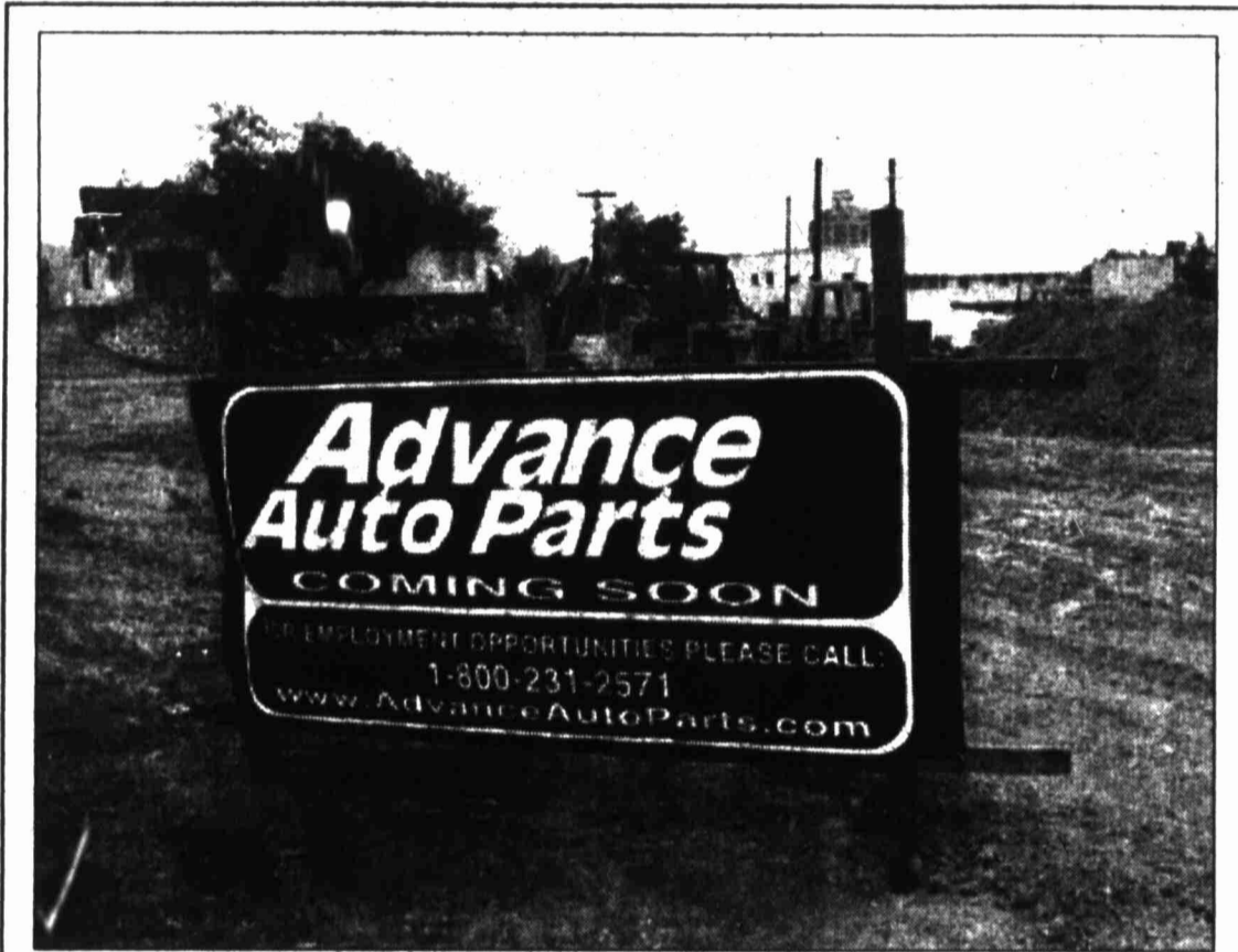
Construction has started on the building for Advance Auto Supply which will be located at the 800 block of Gregg. Several construction projects are currently going on in Big Spring.
