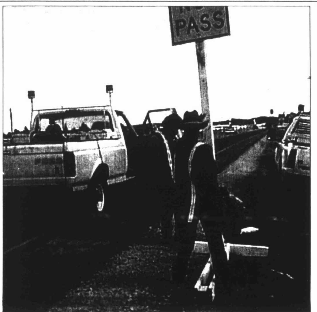
Barricades Unlimited Inc. employees Ruben Castillo, Carlos Adkins and Ruben Nunez of Lubbock put up signs along U.S. Highway 87 warning drivers to slow down for construction work ahead. Work begins Monday on a complete renovation of the roadway from Interstate 20 to Second Street.
