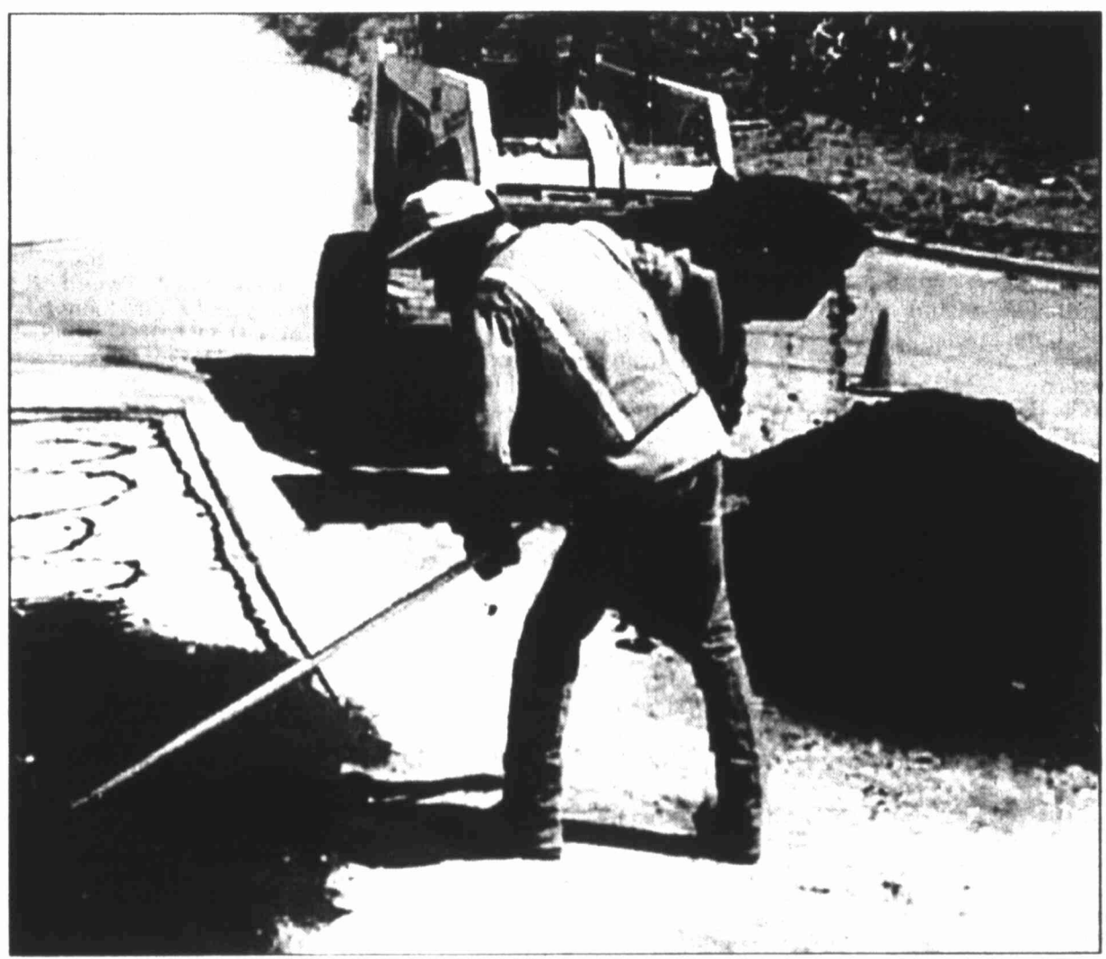
Roy Spivey, with the city street department, applies tack oil to the street at 12th and Main before asphalt is put down.
