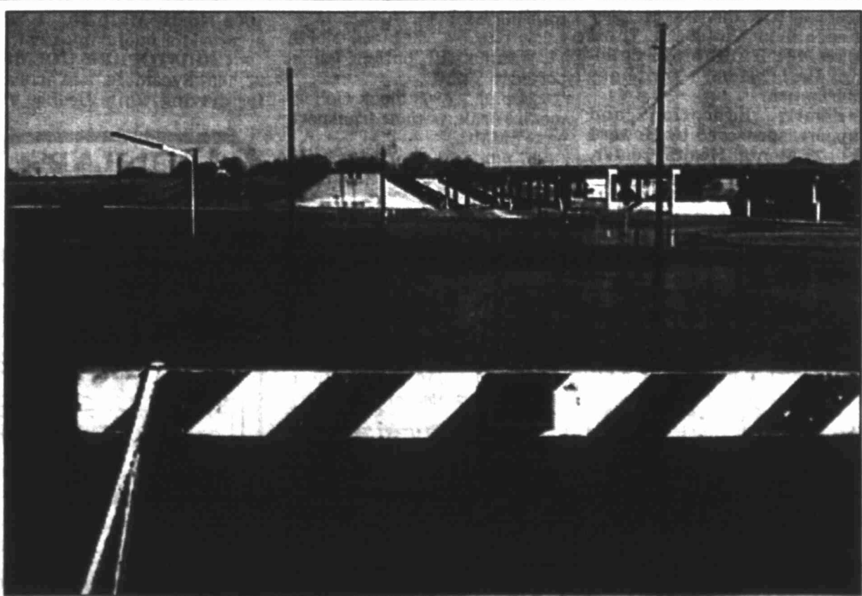
Birdwell Lane was still blocked off today as a result of heavy rains here Wednesday night and early Thursday. The water, overflowing from Beals Creek, was also flooding most of the railroad yard in the downtown area.
