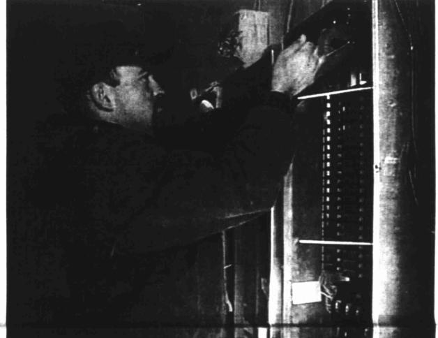
Carey Burchett of B&B Electric installs the breaker box at the new multipurpose center for the SouthWest Collegiate Institute for the Deaf. This construction site will be joined by another project. the diagnostic center, as new facilities on the SWCID campus continue to be created.
