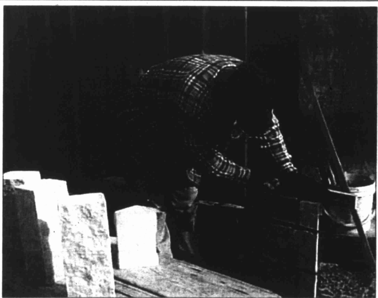
Raymond Lovira of Tall City Masonry out of Midland applies mortar to brick for the new Big Spring Westex Telcom Service Center on Scurry Street. The building is expected to be complete in April.
