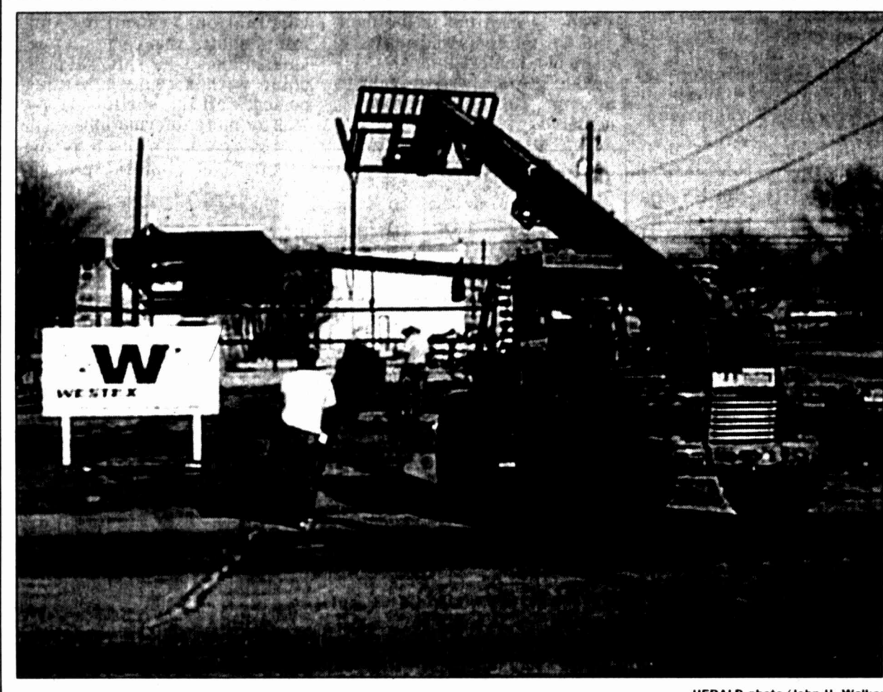
Steel framing is going up on the WESTEX Telecom customer service center on Scurry Street. The company is expanding its digital/cellular and long distance telephone service.
