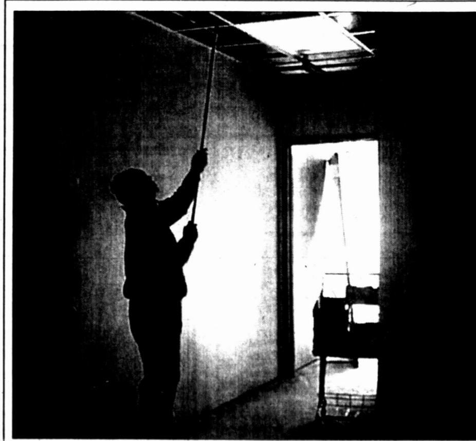
Andrew Agullar, an employee of Woodruff and Rose Construction of Midland, is tying wire in the Trinity Baptist Fellowship Annex. Construction is expected to be finished at the end of this month.
