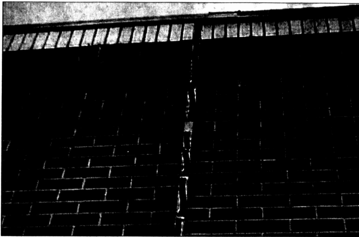
As August came to an end, trustees of the Big Spring Independent School District were considering an expensive, involved process to halt the foundation shift of Big Spring Junior High School, which caused large cracks such as this one in walls and floors.
