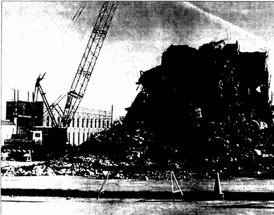
Midwest Wrecking brings down the tower portion of the Permian Building, ending a year-long project in which funds were raised, legal matters handled and a contract awarded for demolition of the aging, downtown structure.
