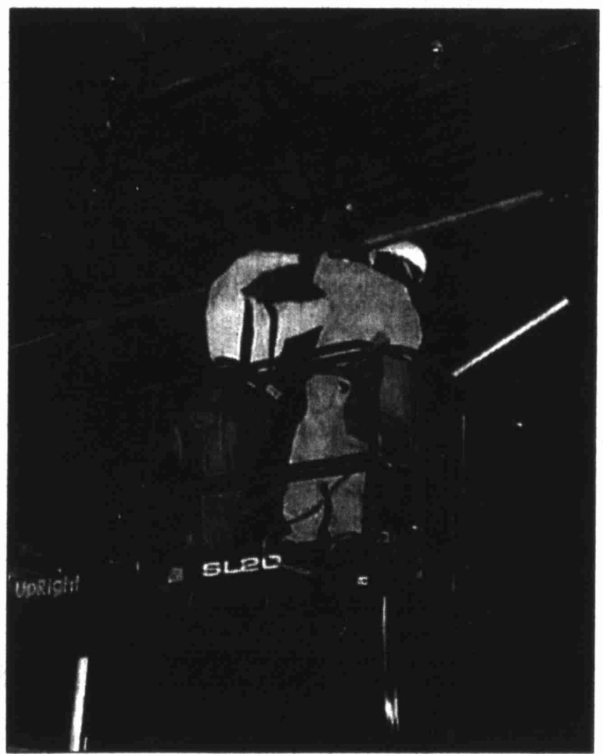
Doug Johnson, left and Larry Loya install conduit for computer cabling during the remodeling of the former TG&Y building into a StarTek USA call center facility in the College Park Shopping Center. The center is expected to open Dec. 1.
