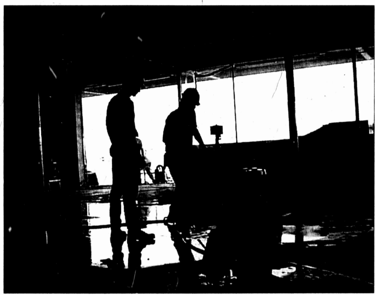
Ben Wehrich of Lee George Construction cuts the floor of the old Furr's store on 11th Place today while Steve Wells supervises. The 22,000 square-foot building, vacant for several years, has been purchased by Trinity Baptist Church and is being remodeled for classrooms and a fellowship hall.
