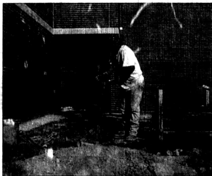
Ugo Quintana, a workman with Hayward Baker, Inc. of Dallas, cleans drilling pipe in preparation for continued compaction grouting work to stabilize the sinking southeast corner of Big Spring Junior High School.
