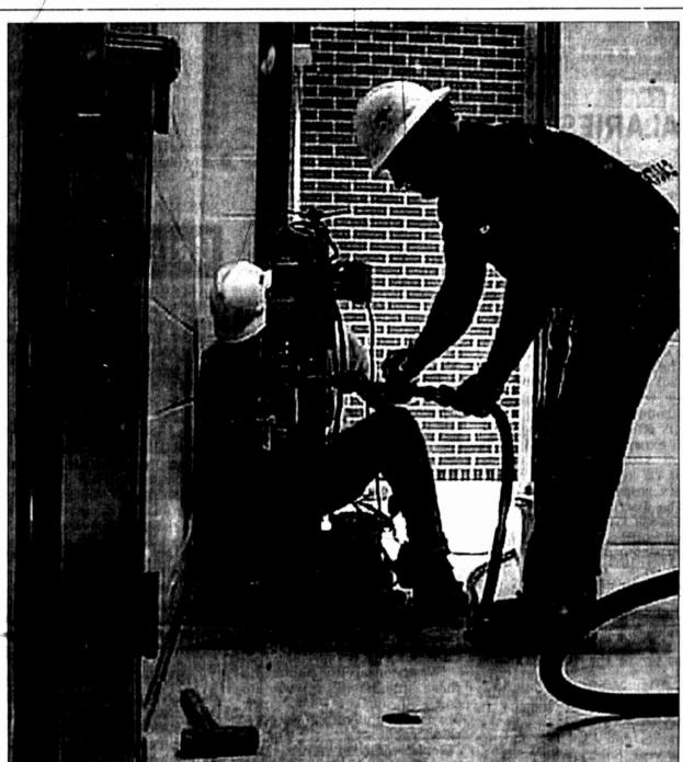
Compaction grouting work has begun on Big Spring Junior High School. A crew from Haywood Baker of Dallas began drilling holes in the terrazzo flooring at the southeast corner door today. Compaction grouting involves pumping concrete under the building to stabilize the soil to stop the sinking and wall cracking the \$10 million new school has experienced. Drilling is Chris Fletcher, supervised by Corey Shipwash, right.
