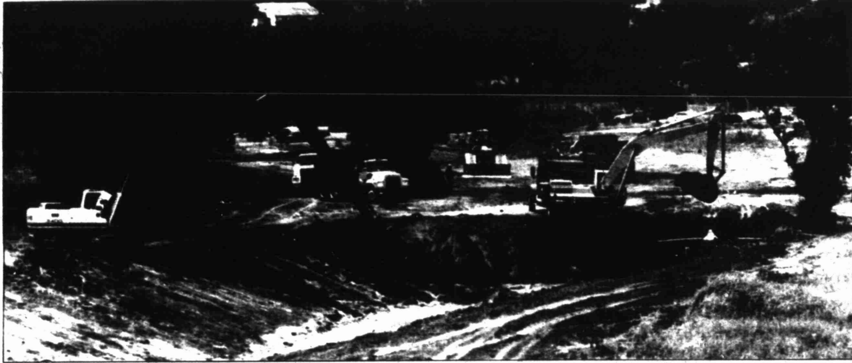
Beals Creek has been the subject of a $10,885,800 construction project that includes 7,280 foot of channel that measures about 20 foot across the grassy bottom, and between 100 and 200 feet at the top.
