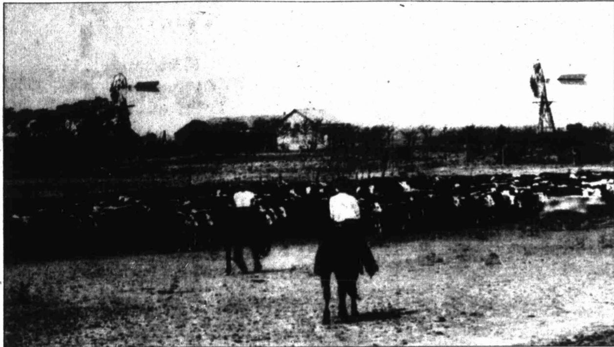
Cattlemen early learned that they had to adapt to the country, otherwise they would be broken by it. During the first quarter of century for Howard County there were at least two, and possibly three, severe droughts.
