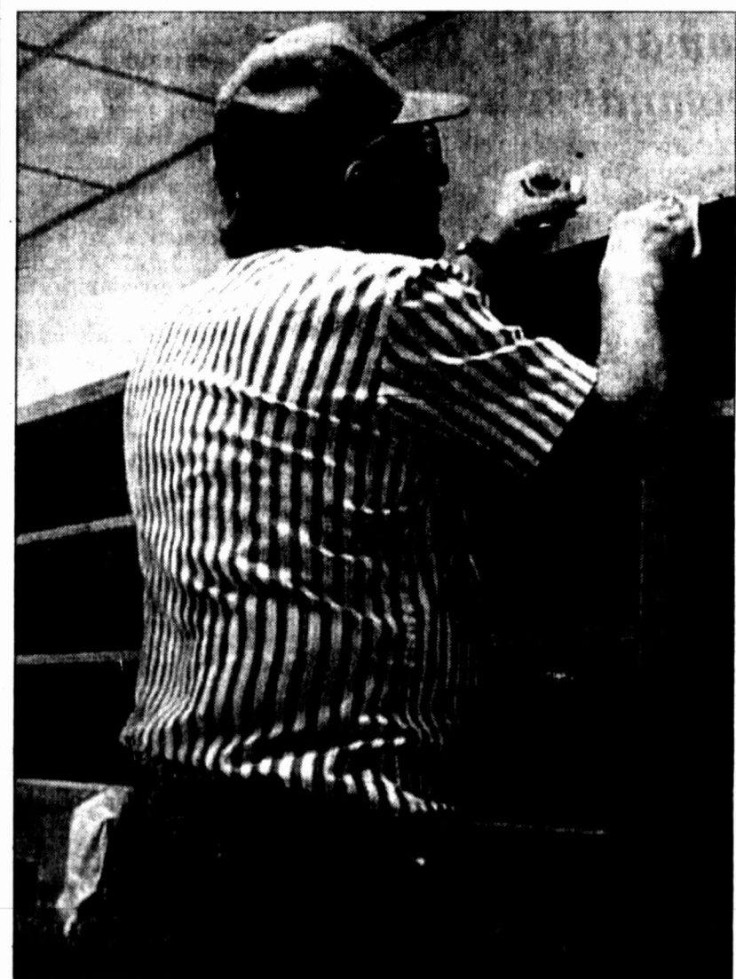
Earl King of Monterey Construction does the finishing work to cabinets in one of the classroom storage areas at the new Big Spring Junior High School.
