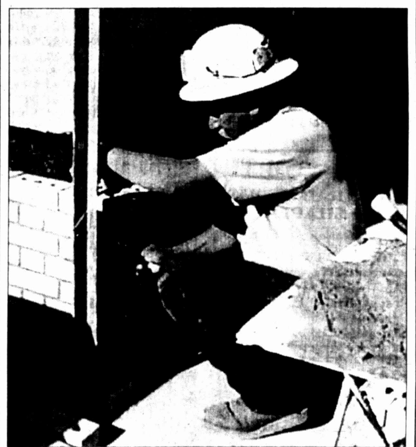
Poly Castaneda of A-Aguirre Construction in Big Spring finishes the mortar and brick work on the external areas of the expansion at the VA Medical Center. The exterior is expected to be complete this week.
