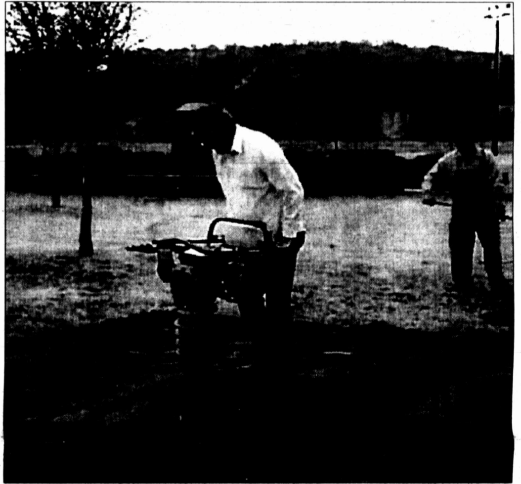
HERALD photo/John H. Walker Pat Carnahan (foreground) and Danny Kennedy work to prepare the site where the chapel will be constructed at the Vietnam Memorial. Carnahan is operating a compactor to pack the dirt where the concrete pad will be poured.
