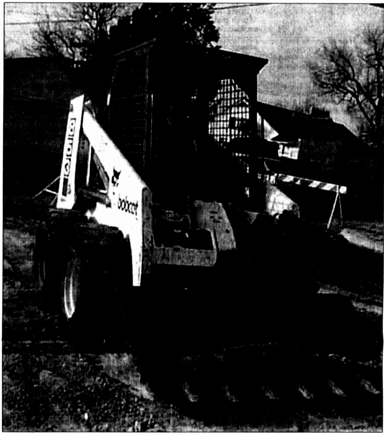
Mike Coffman uses a Bobcat to help make water line repairs in the vicinity of Runnels and 18th Street this morning.
