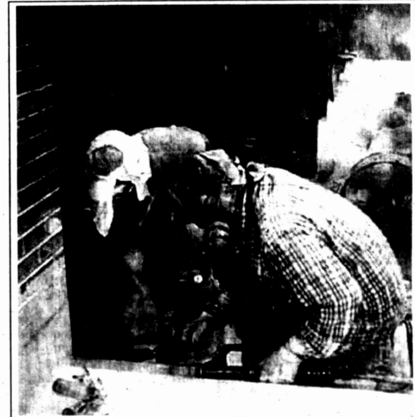
The air is filled with white chalk as Mark Zanchettin, left, and Chris Scott, sand the terrazzo poured onto the steps in the mall area of the new Big Spring Junior High School.
