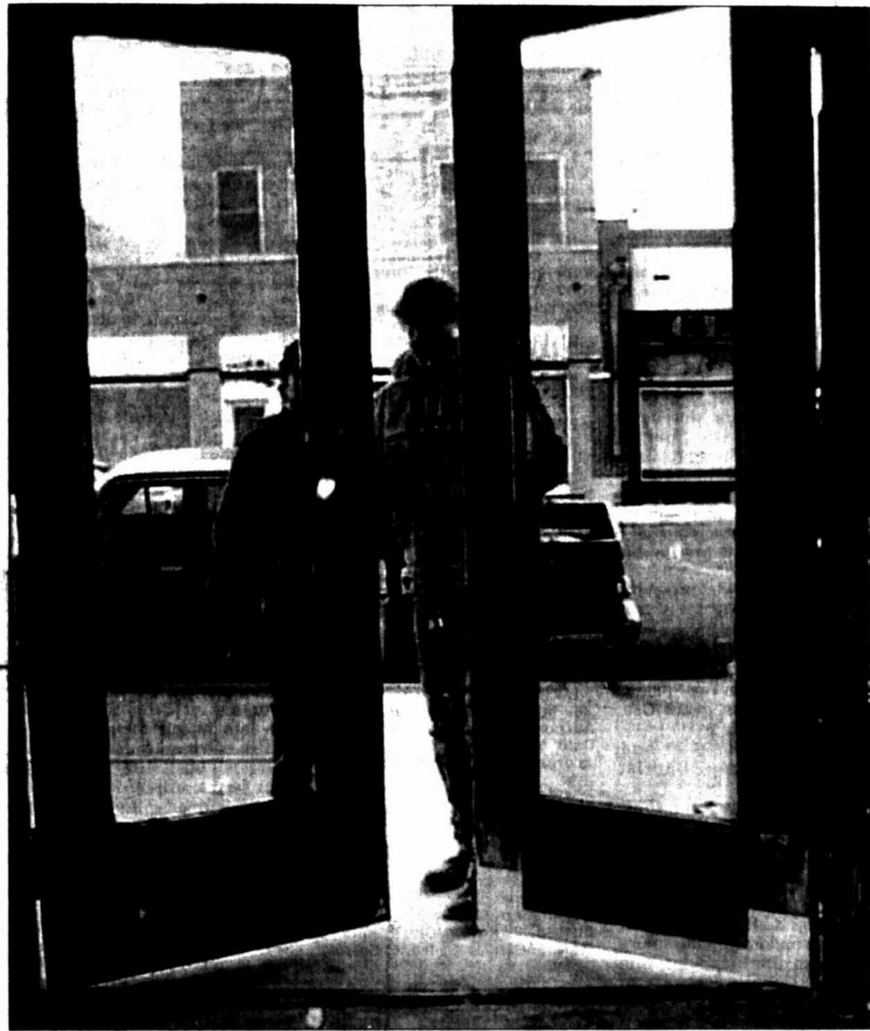
Chris Abshier, center, and Terry Sawyers of Bob's Custom Woodwork check the balance of the newly hung glass doors at the Settles building on Friday. The doors were removed to be resized and fitted with new glass panels.
