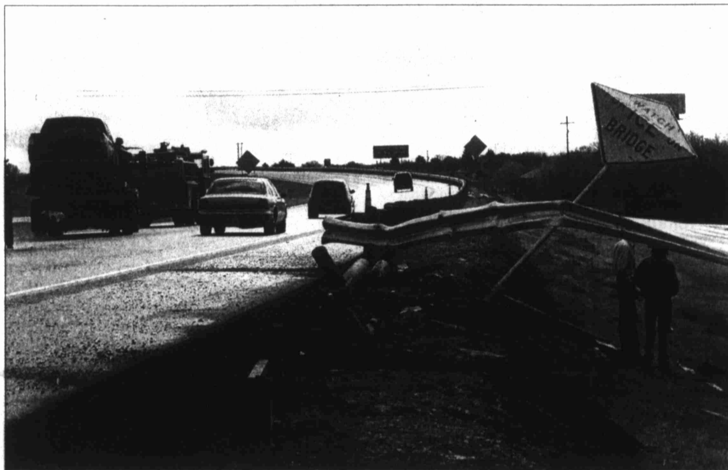
Highway department workers examine a twisted section of guardrail at the 178 mile marker of Interstate 20 Tuesday morning. The guardrail was damaged when it was struck by a Ford pickup. No other details of the accident were available at press time.
