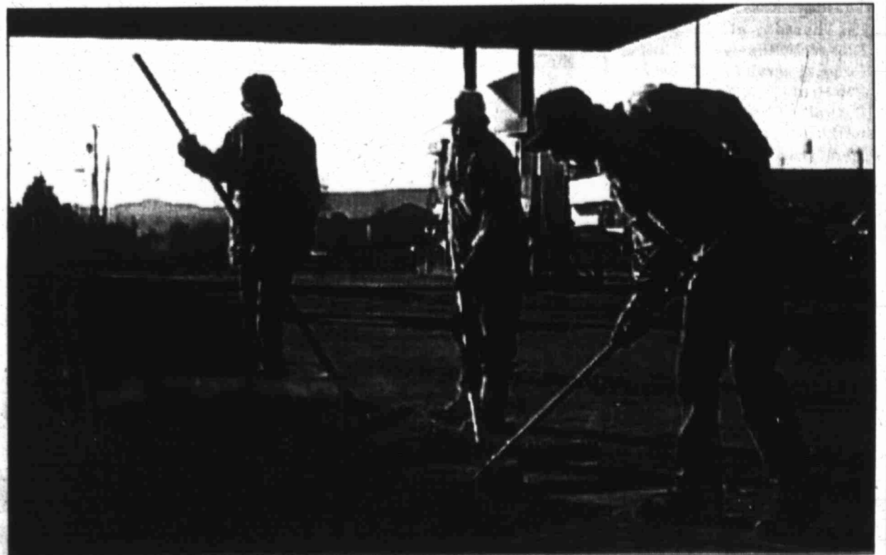
Cline Construction employees (from left) Steve English, Joe Torres, and Mitch Gutierrez put the finishing touches on the parking lot of Kates Fina Mart following the removal of several underground storage tanks.
