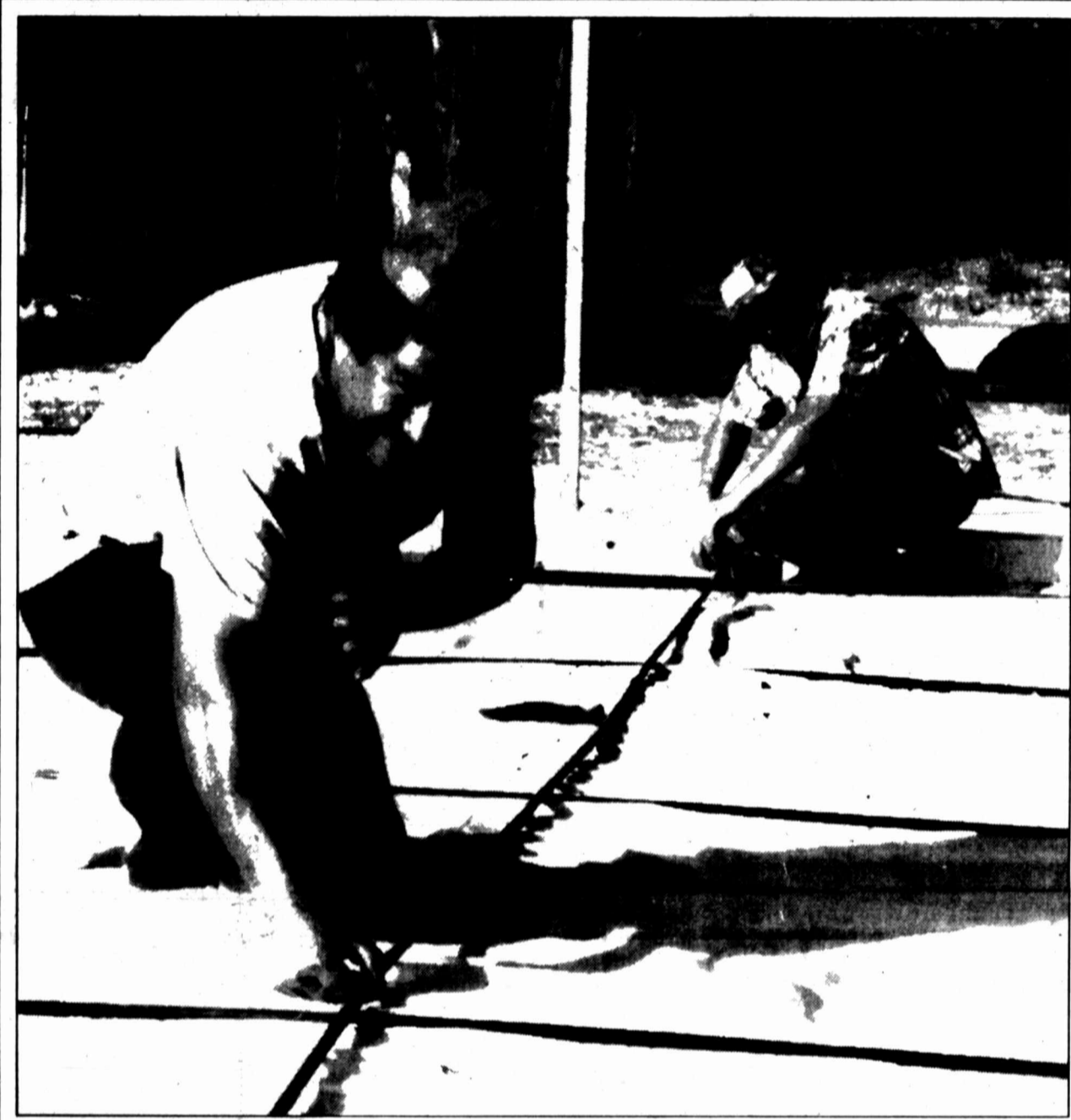
HERALD photo/Linda Choate Tony Mata, left, and Mack Leal are part of the construction crew conducting resurfacing work at the Figure 7 tennis courts at Comanche Trail Park.
