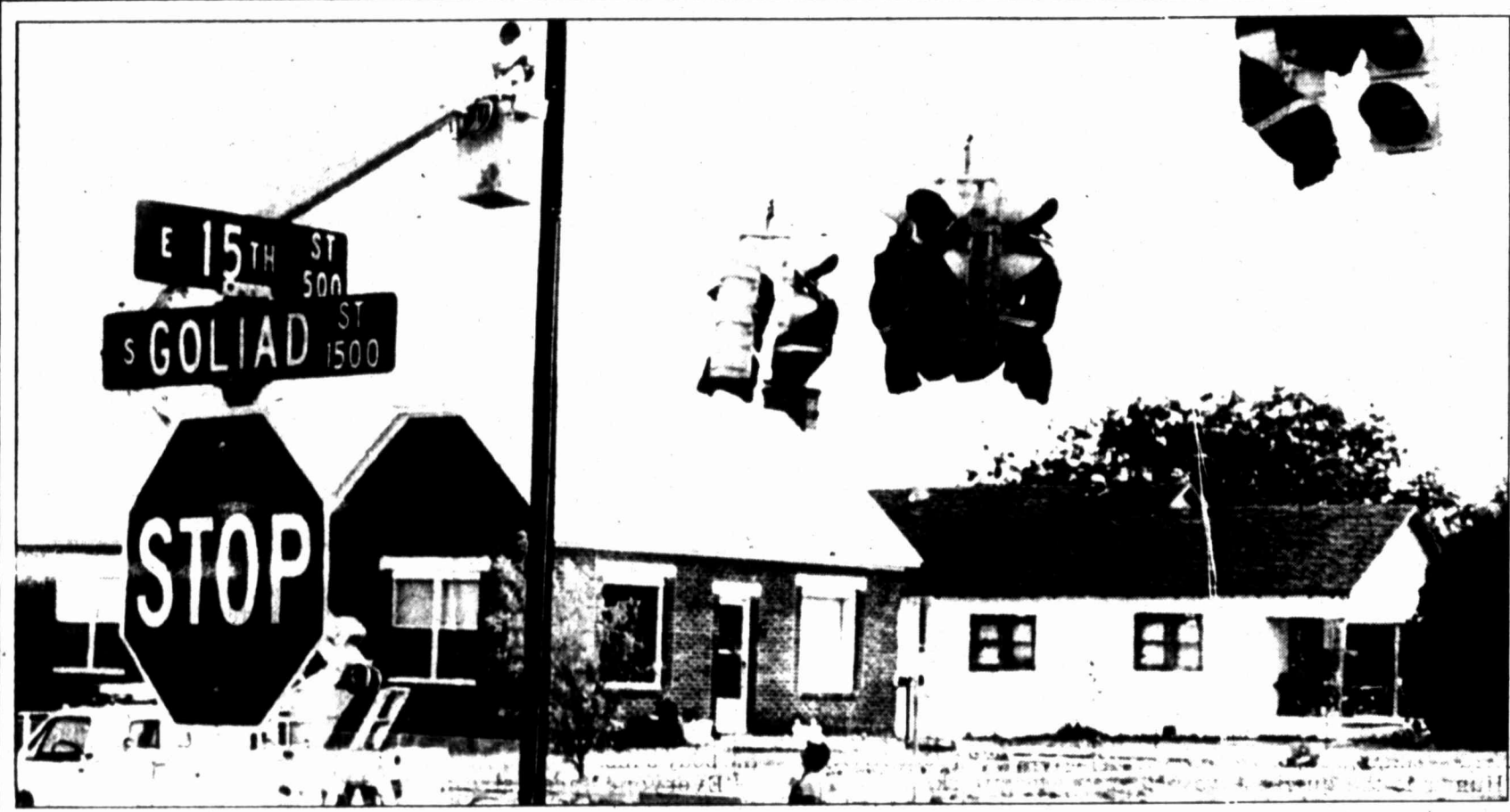
City of Big Spring employees Bobby Davis (in utility bucket) and Joe Arnold make adjustments to a new traffic signal at 15th and Goliad. The new signal is expected to start operating in about three weeks, when more wiring and some testing is complete.
