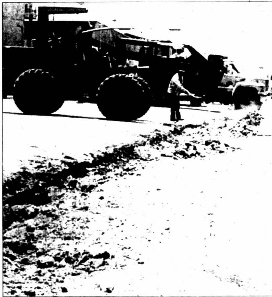
City workers Jurge Parra and Raul Martinez work on replacing a sidewalk and curb after water line replacement last week. The city spends between $300,000-500,000 a year on water lines and filters.
