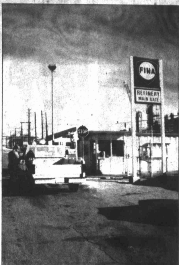
Plant Entrance Fina Refinery.
