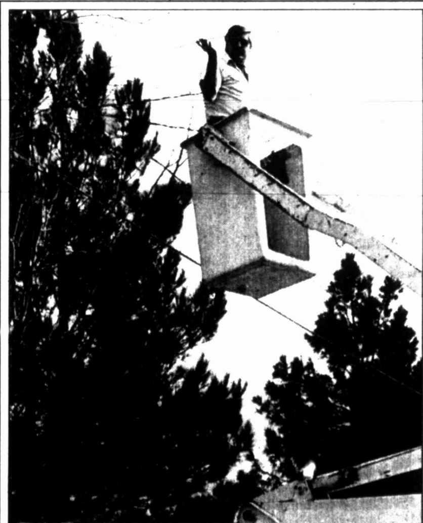
Steve Westbrook of TCA Big Spring Cable TV avoids some power lines as he makes an installation call recently.
