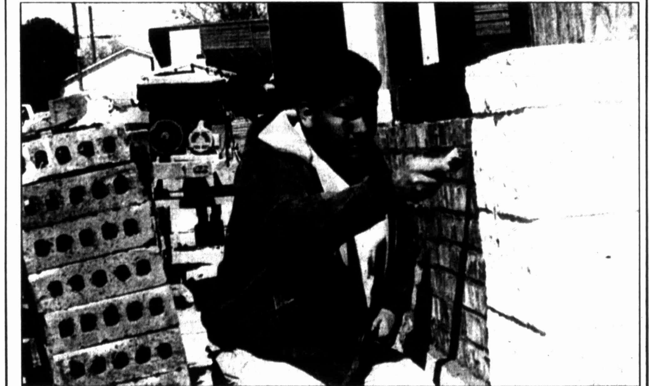
Lee Balderas is putting some finishing touches on the brick work of the Schlotzky's sandwich shop, scheduled to open in Big Spring around March 15. Schlotzky's is expected to initially hire 40 employees and retain at least 25 employees once the store is fully operational.
