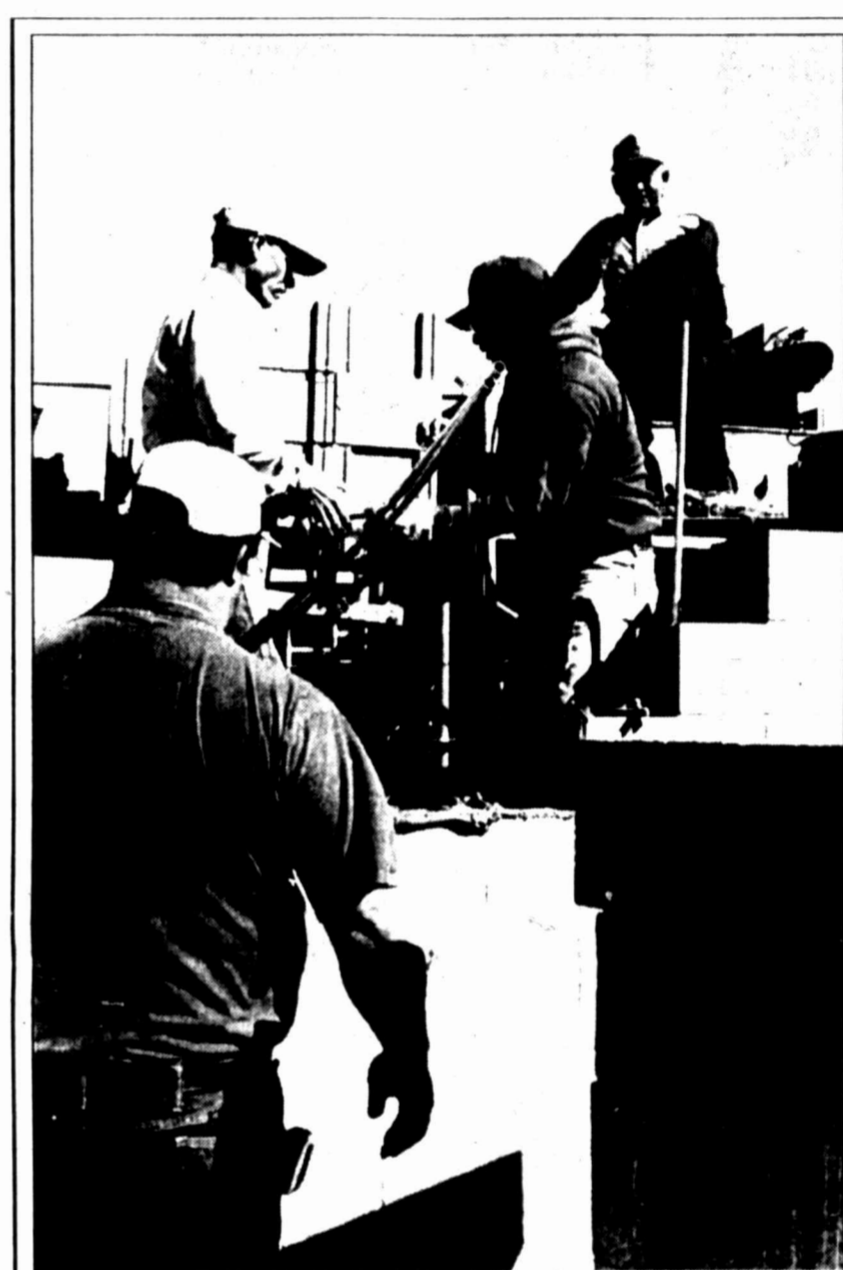
Progress continues on SWCID addition as Southwest Masonry workers Bobby Willis and Hermelio Bital (center) construct the outer wall.
