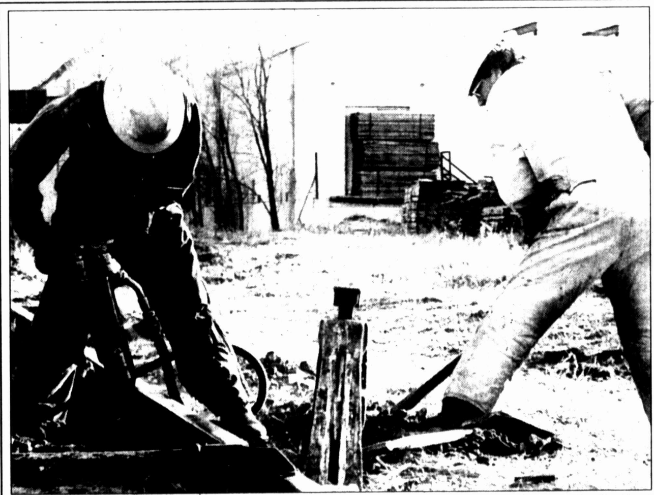
HERALD photo/Jonathan Garrett Fidel Ruiz pries up a tie as Jorge Ruiz drives a railroad spike into it to connect the rail on Wednesday. Trac-Work Inc., out of Amarillo, expect to be finished with the work by mid-February.
