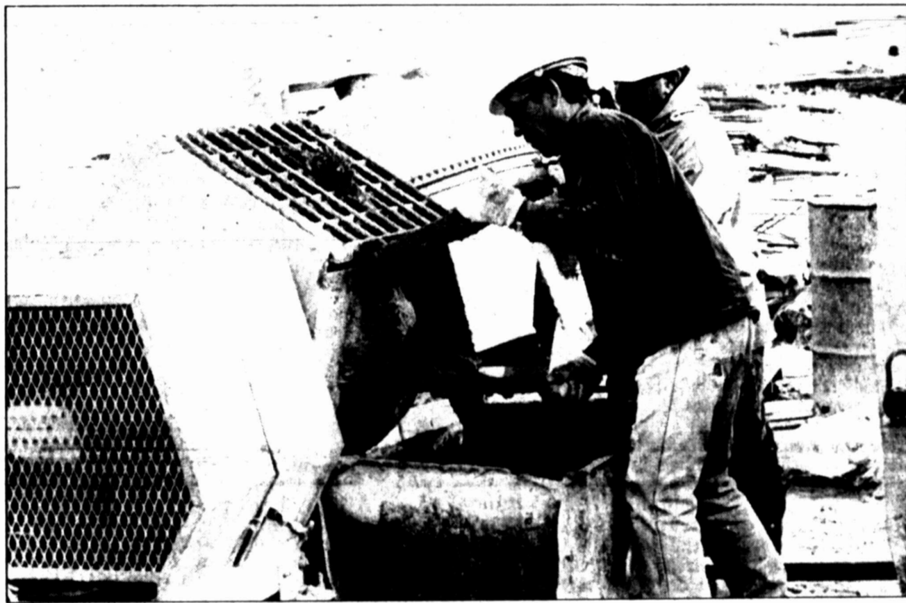
Felipe Hernandez (left), with J & E Masonry, and Andy Rodriguez, with Monterey Construction, pour mortar into one of the containers used to transport it to the various location it is needed.
