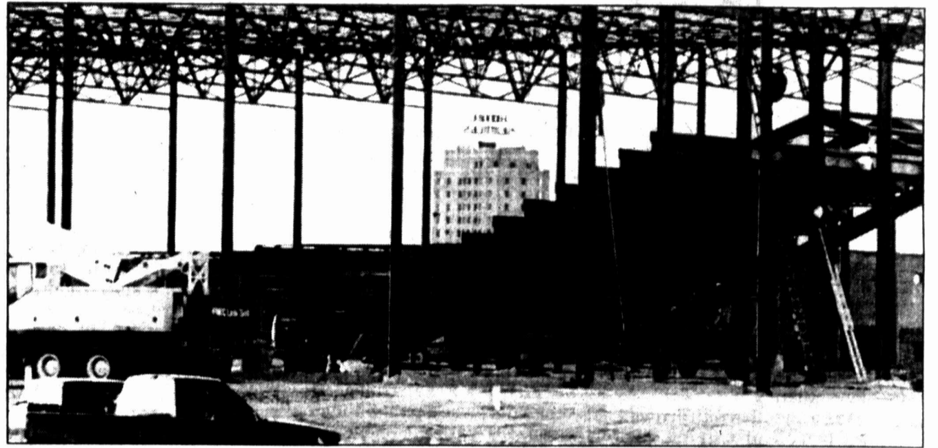
The Settles building is visible through the steel of the superstructure at the new junior high school. In this photo, steel beams are being erected for the seats in the gymnasium.
