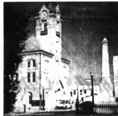
The opera house in Newberry, S.C. is being restored.
