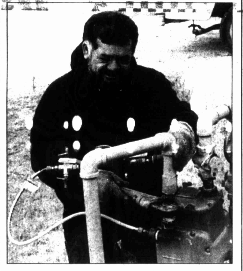
Pete Hernandez with Energas was doing pressure testing Tuesday on gas lines to insure that they are ready for the extra demand of the winter months.
