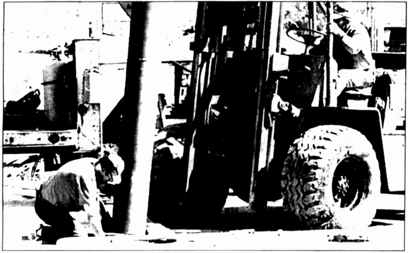
Workers install the pole that will support the new canopy at Neighbors Convenience Store at 3315 E. FM 700. Owners Alan and Della Partee are adding the canopy and new gasoline pumps for the convenience of their customers.
