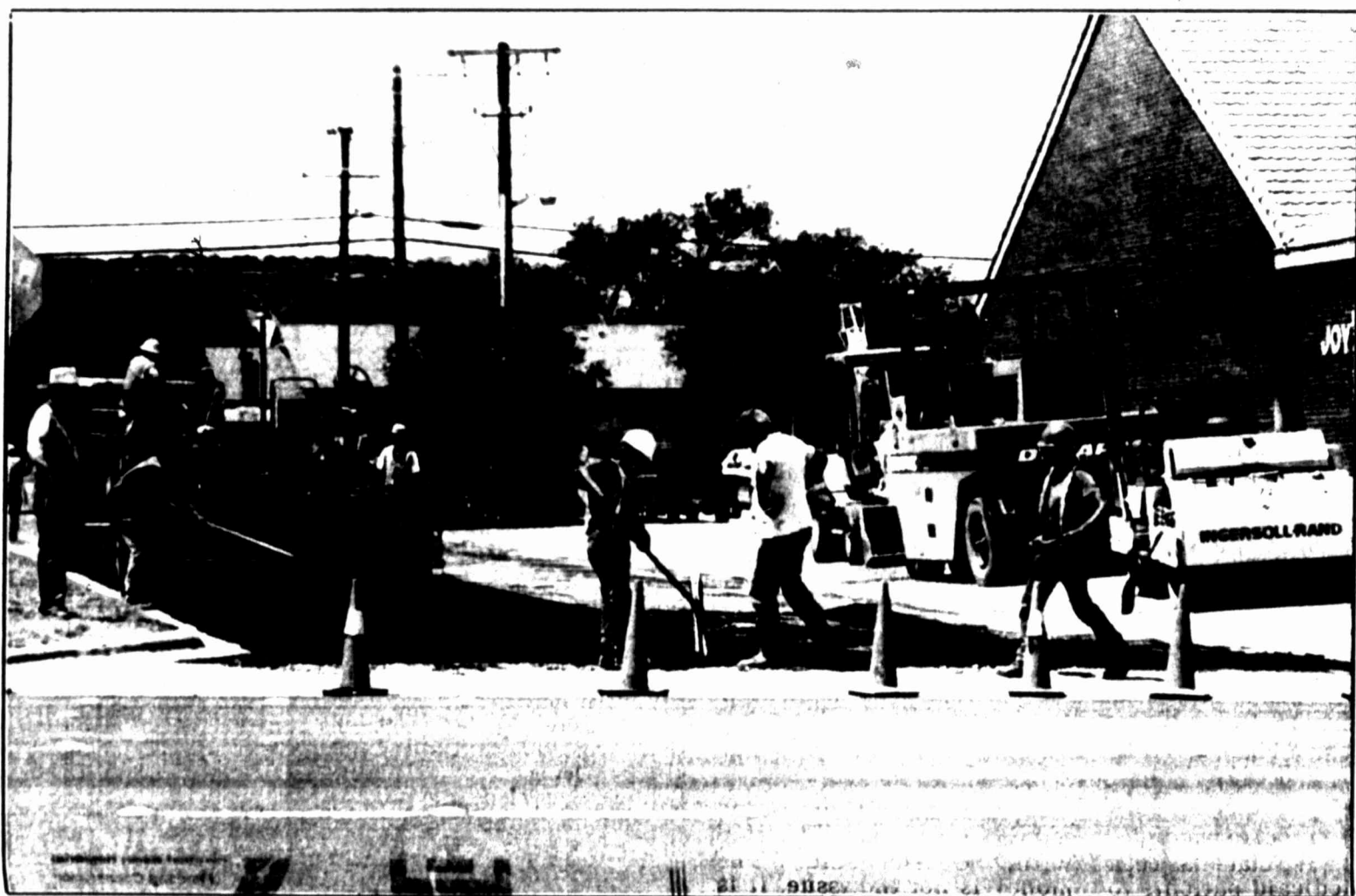
City crews continue putting a new look on several city streets by either sealcoating or totally rebuilding them. This stretch along 21st Street between Joy's Hallmark and H-E-B is being sealcoated. Several other streets will be worked on in the next few weeks.
