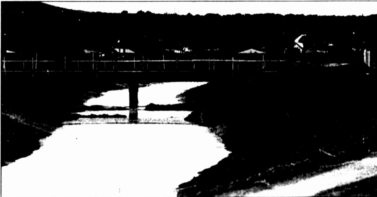
HERALD photo/Jonathan Garrett The Beals Creek Flood Control Project got a brief test Sunday afternoon after heavy rains over a short period of time resulted in a heavy runoff. Shown in the photo is a new bridge constructed in the vicinity of the old roundhouse, northeast of the engine fueling depot.
