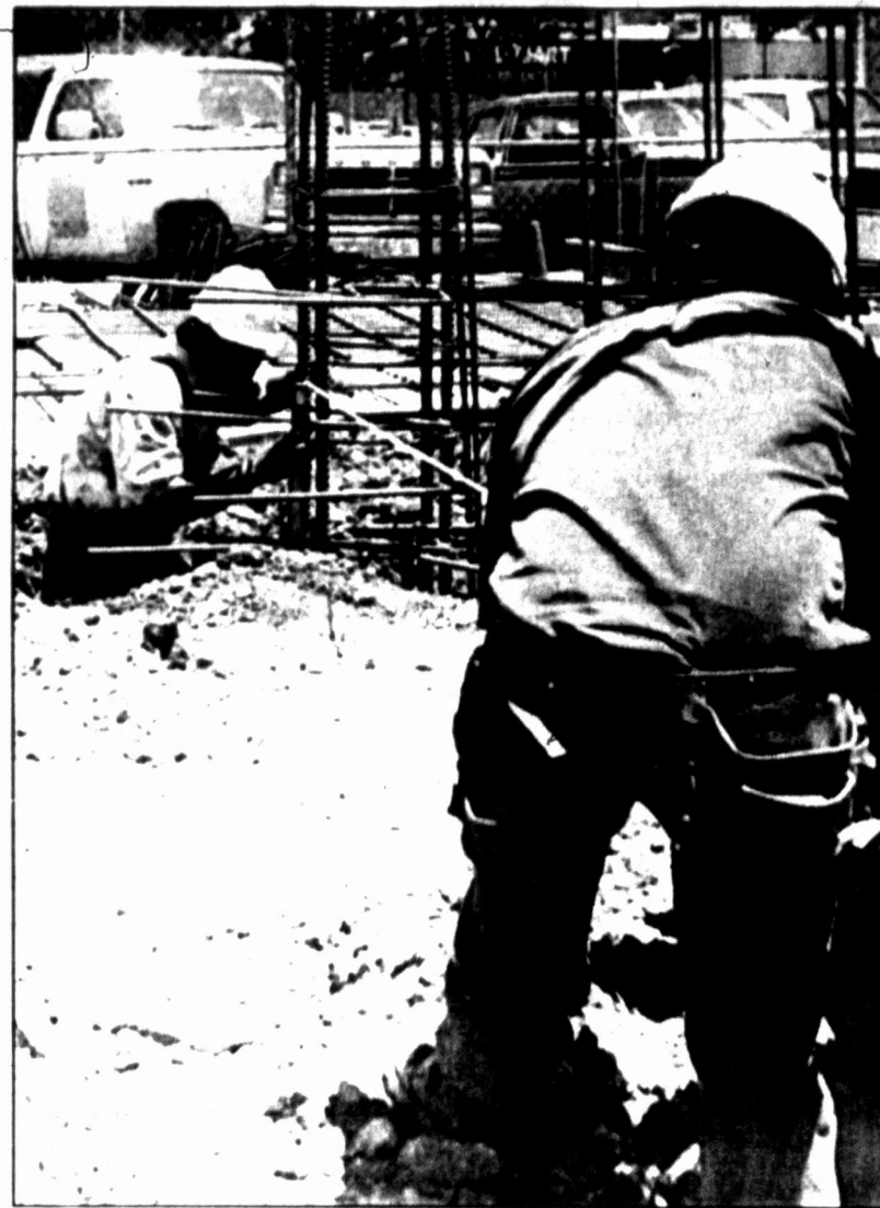
HERALD photo/Jonathan Garrett Catarino Ornelas (left) and Leo Calderin measure the distance from the wall to the support pillar of what will be the clinic at the Veterans Administrative Hospital. Construction is expected to be complete in nine months.
